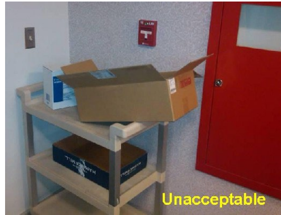
Obstructed Manual Pull Station
